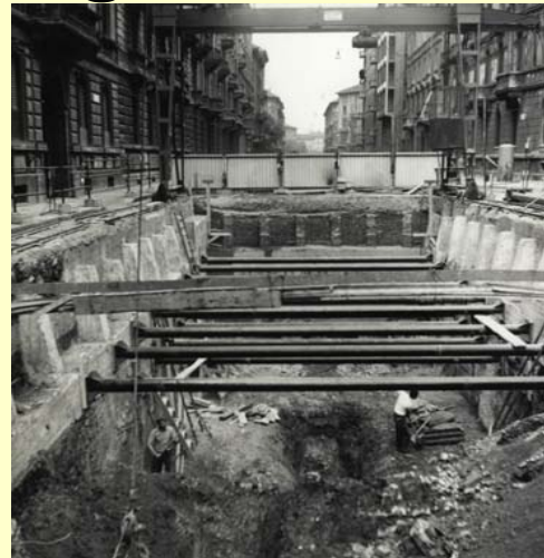
Scavo in trincea – Cut and cover (cuci e scuci o sistema Milano )
